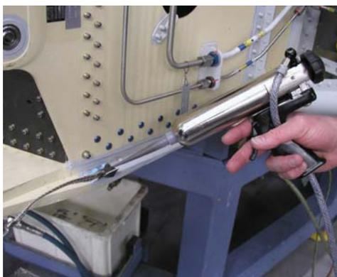
*Applying mixed sealant from a cartridge gun*
